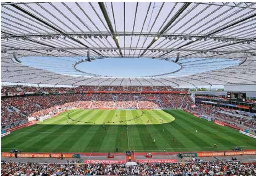
*The BayArena, home of the German soccer team Bayer 04 Leverkusen. A polycarbonate roof is noted for its high break resistance, impact strength, temperature resistance and light weight.*
